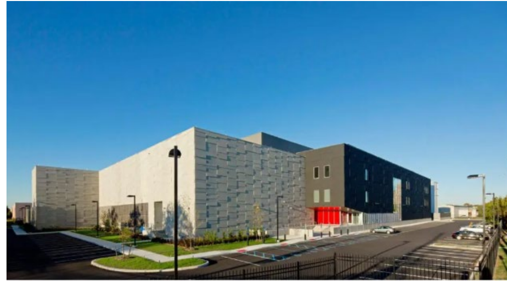
Colocation Data Center – Equinix at 800 Secaucus Road, Secaucus, New Jersey. Source: Equinix.
