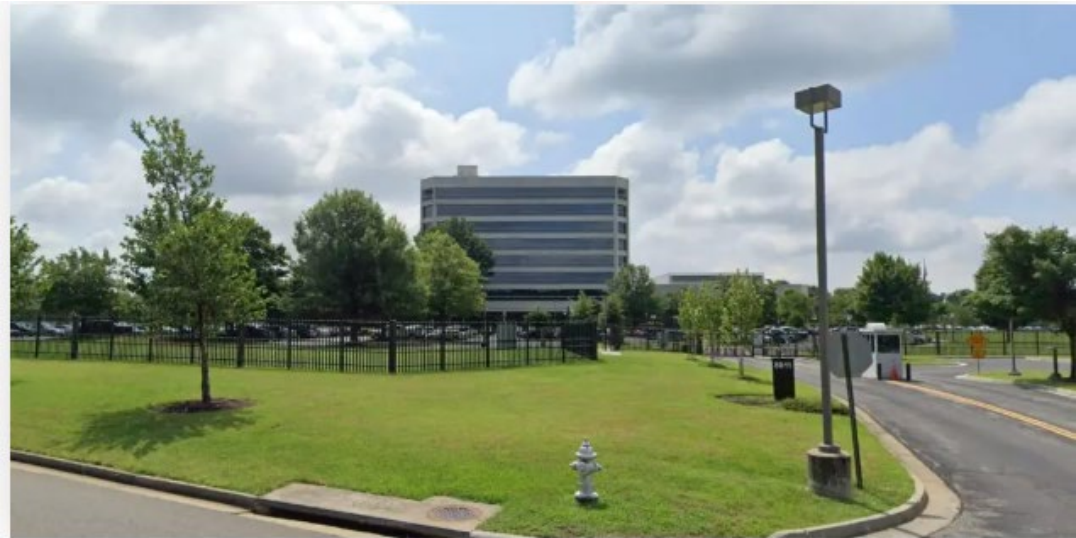
Enterprise Data Center – Bank of America at 8011 Villa Park Drive, Richmond, Virginia.
