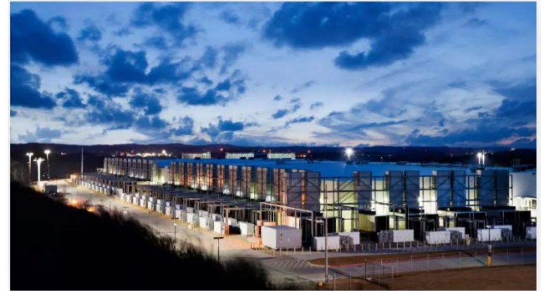
Hyperscale Data Center – Google in Lithia Springs, Douglas County, Georgia. Source: Google.
