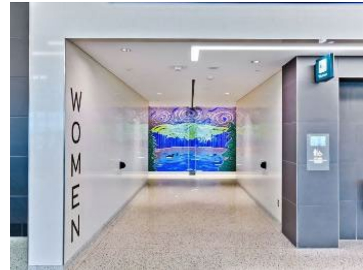
Terminal 2 Restroom renovations; MSP Airport, MN
