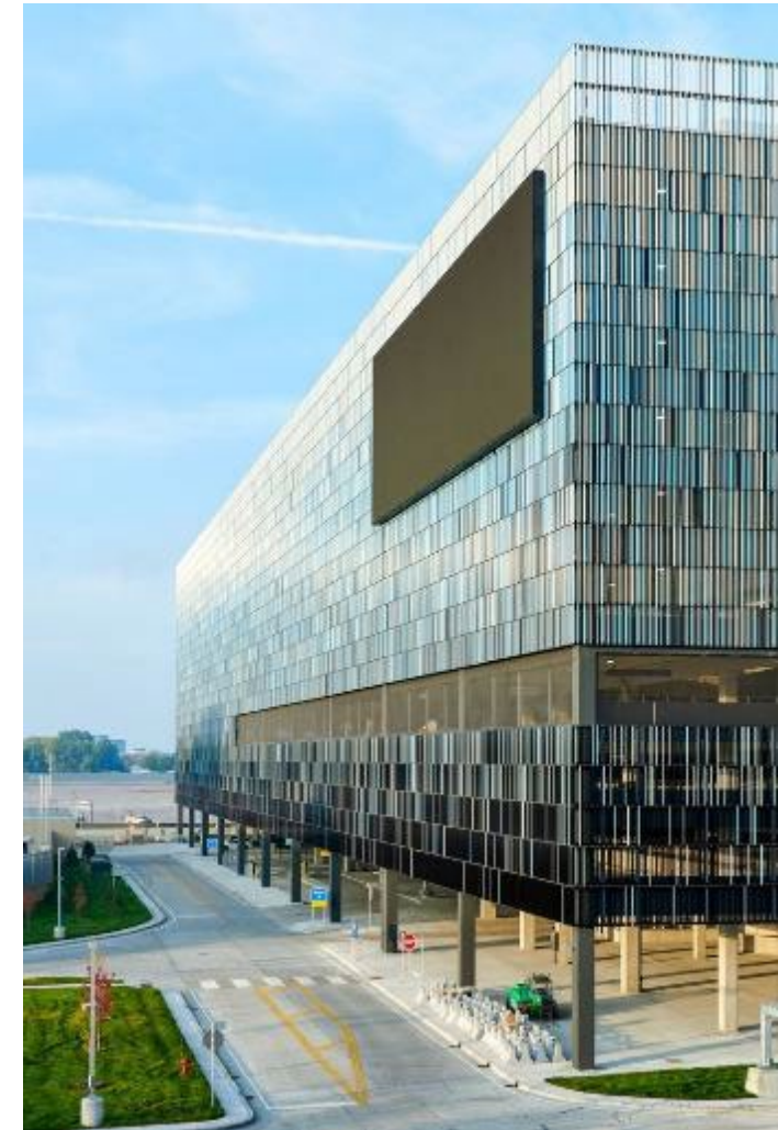
Terminal 1 Silver Ramp Transit Center, MSP Airport
