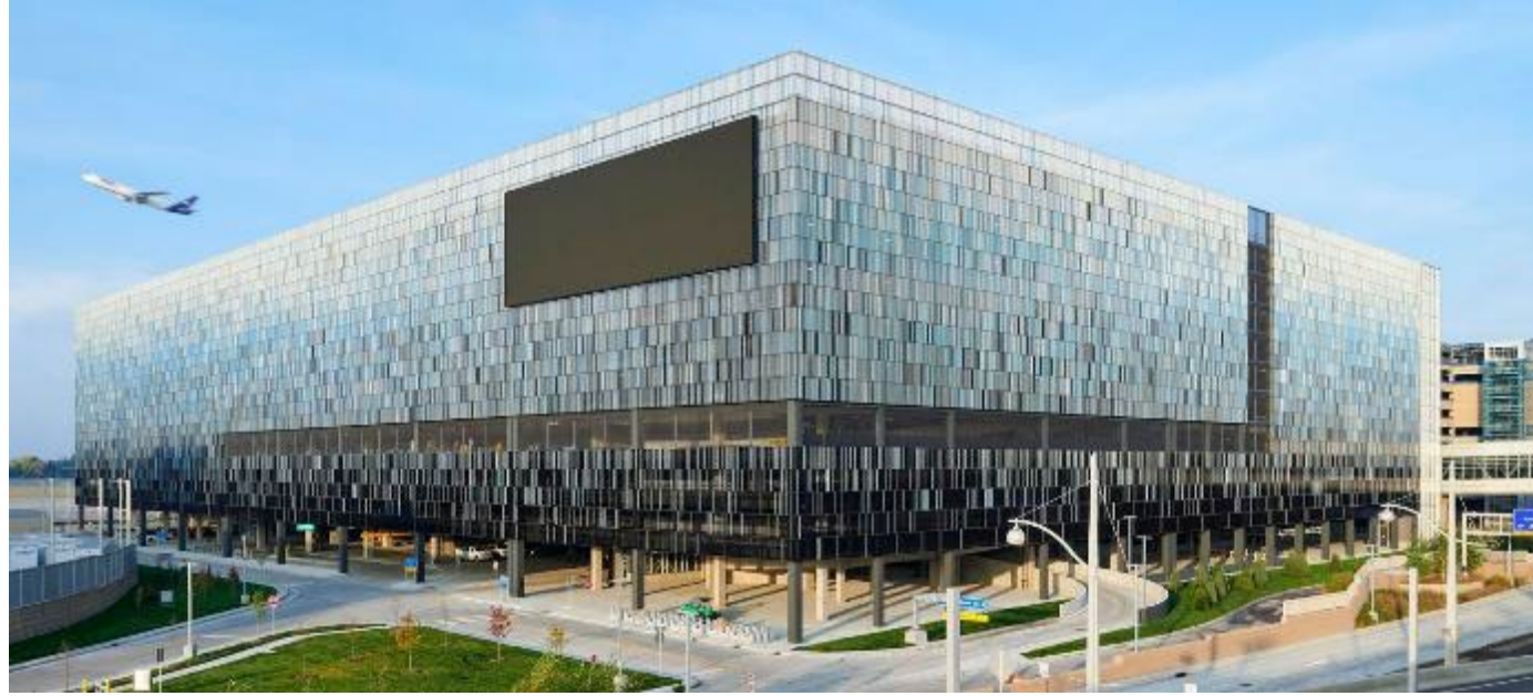
Terminal 1 Silver Ramp Transit Center and Parking; MSP Airport, MN
