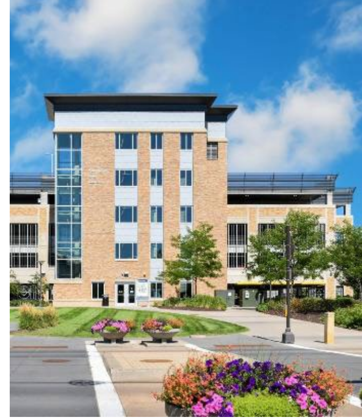
Northstar CRTV Parking Facility, Anoka
