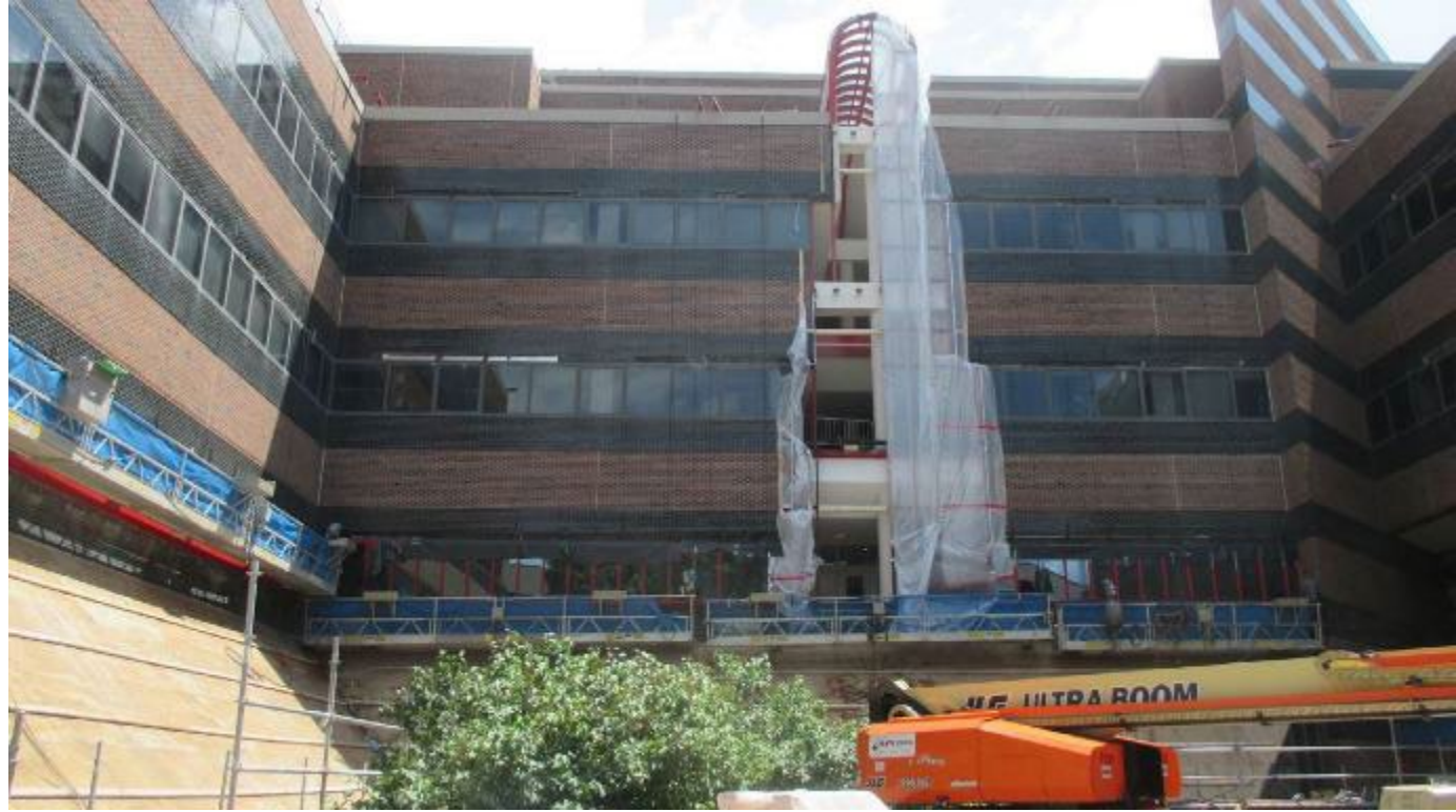
Keller Hall Exterior Envelope Rehabilitation, University of Minnesota
