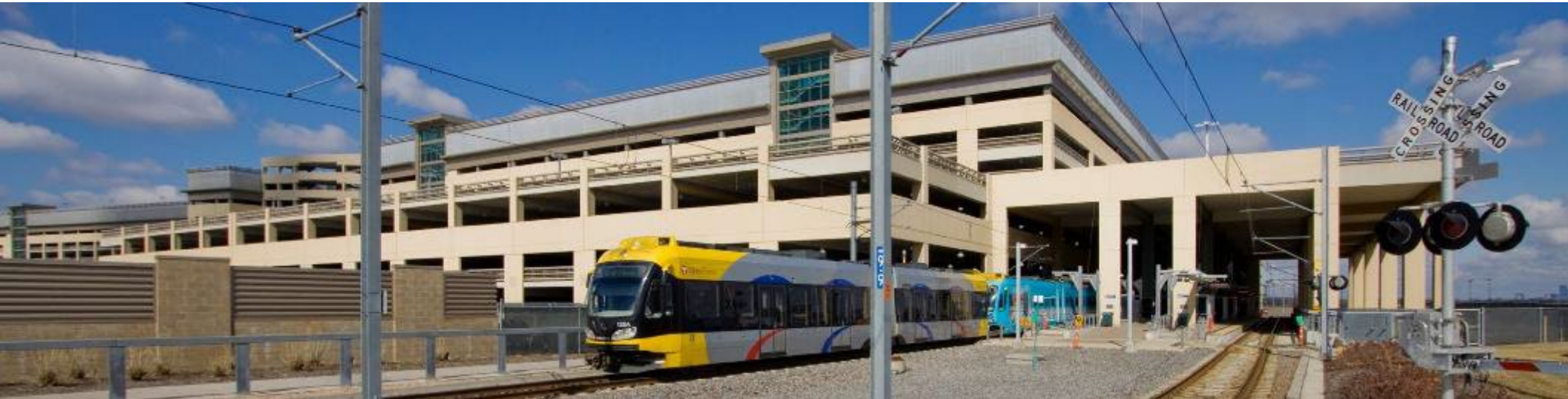
Terminal 2 Parking Ramps and METRO Blue Line LRT Station; MSP Airport
