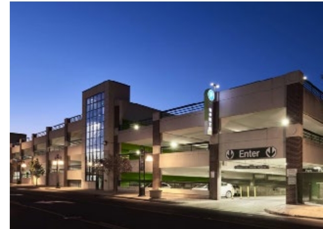
50th and France Ramp, Wayfinding, and Streetscape Renovation; Edina, MN
