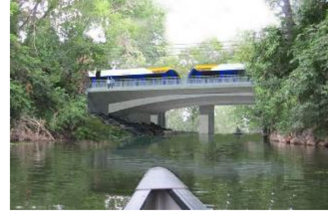
METRO Green Line LRT Extension, Kenilworth Bridge
