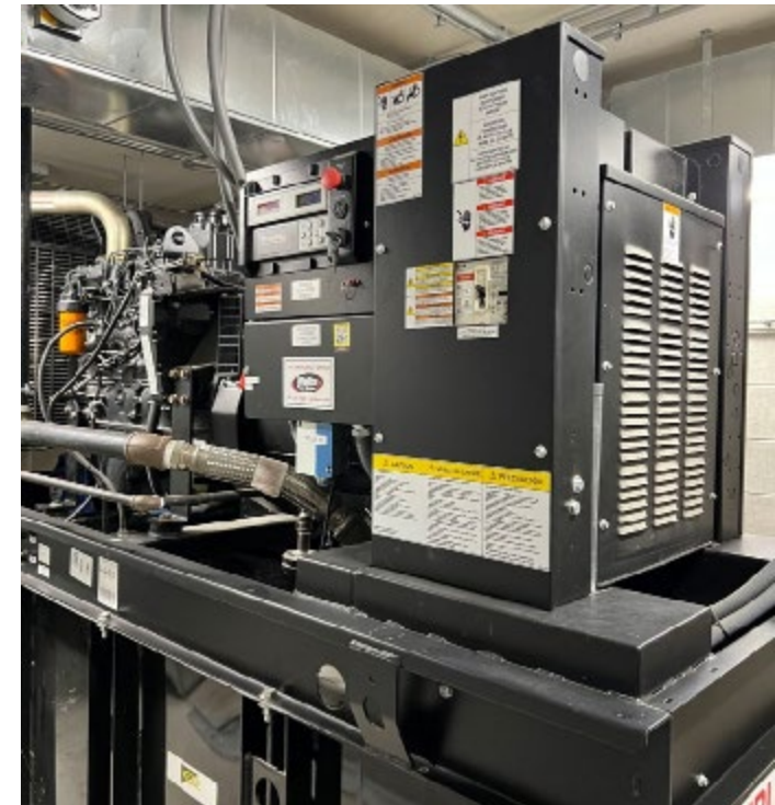
Parking Garage Assessments - UW Madison; Madison, WI
