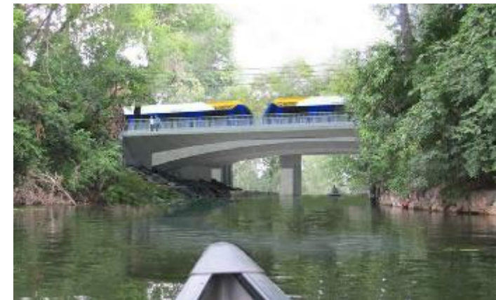
METRO Green Line LRT Extension, Kenilworth Bridge
