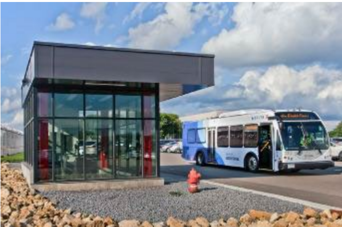
Employee Bus Shelters, Delta Air Lines; MSP Airport, MN
