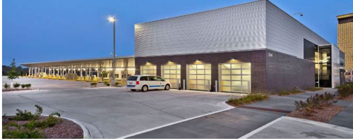
Parking Management Building, MSP Airport
