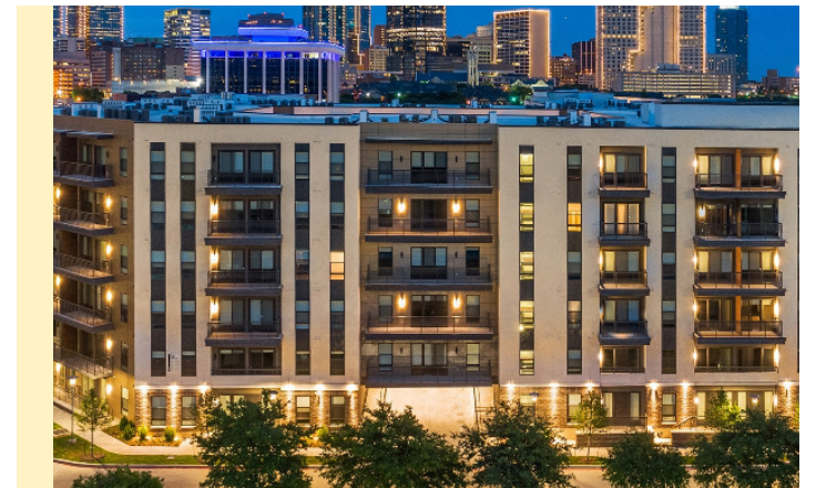
Alliance Development - Fort Worth, TX
