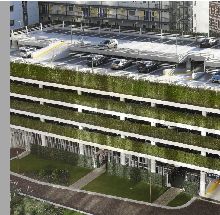
Parking Ramp - Rotterdam, Netherlands
