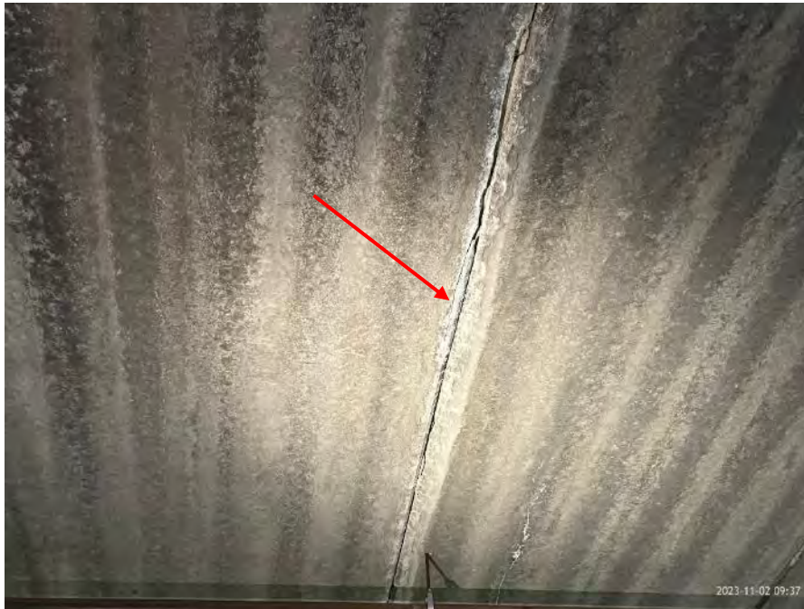
Photo 26 – Example of typical concrete chip/spall (red arrow) at precast plank joint.
