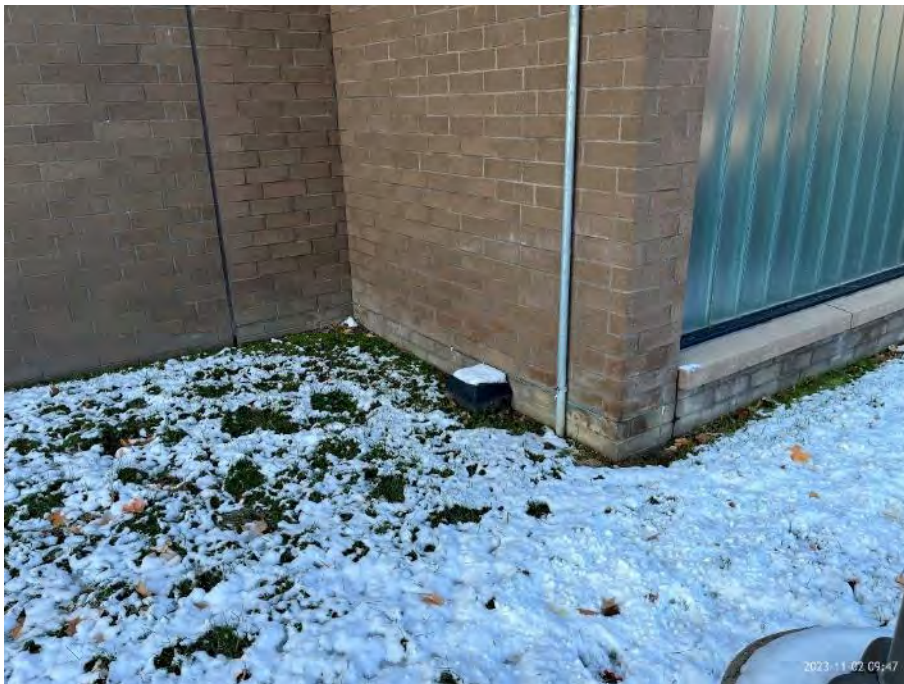
Photo 2 – Exterior of Stair 'E' looking southwest.
