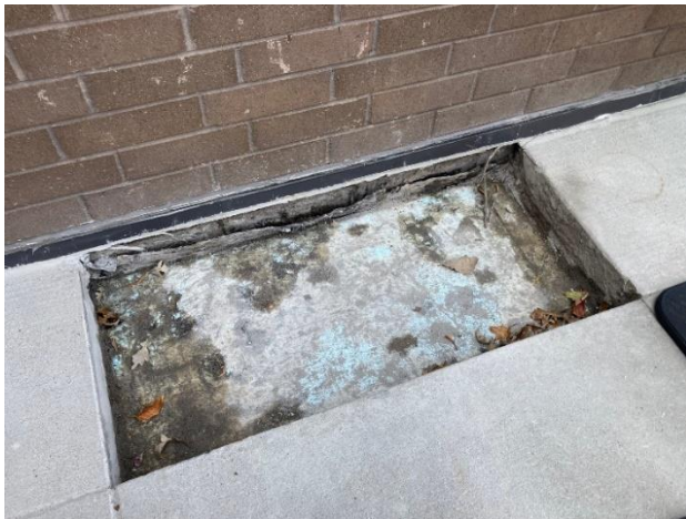
Figure 17: Destructive Test Opening 4 Overall.
