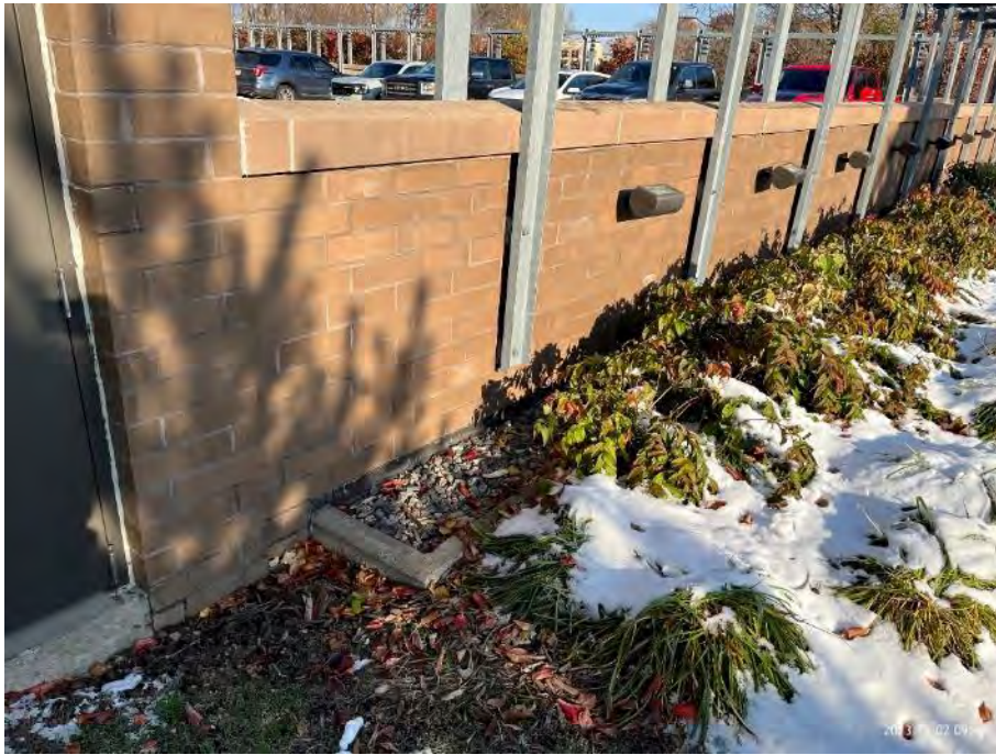
Photo 15 – East side of trellis wall along Grid C.9, looking northwest.
