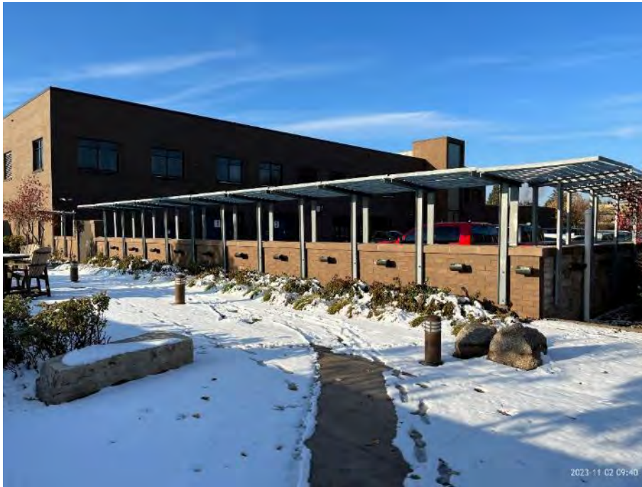
Photo 13 – Overview of patio (formerly green roof) and trellis wall, looking southwest.
