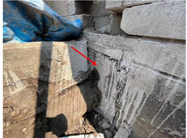
Figure 10: Plaza waterproofing up-turn at CMU starter course.
