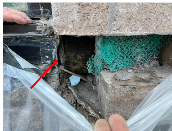
Figure 13: West edge of Stair E window, through wall flashing membrane end.
