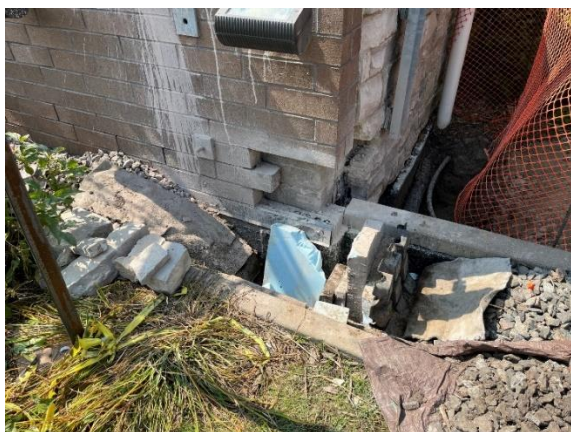
Figure 1: Destructive Test Opening 1 overall.
