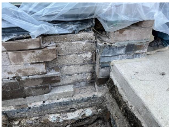
Figure 12: Destructive Test Opening 3 at Stair E.
