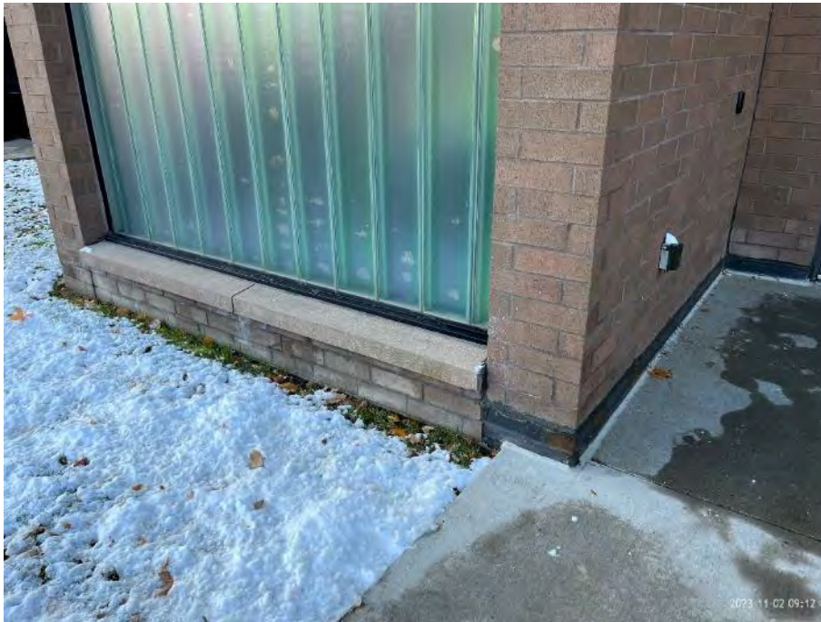
Photo 1 – Exterior of Stair 'E' north and west elevation, looking south.
