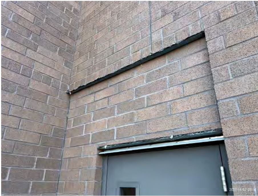
Photo 7 – Lintels, thru-wall flashing, and weeps above service door.
