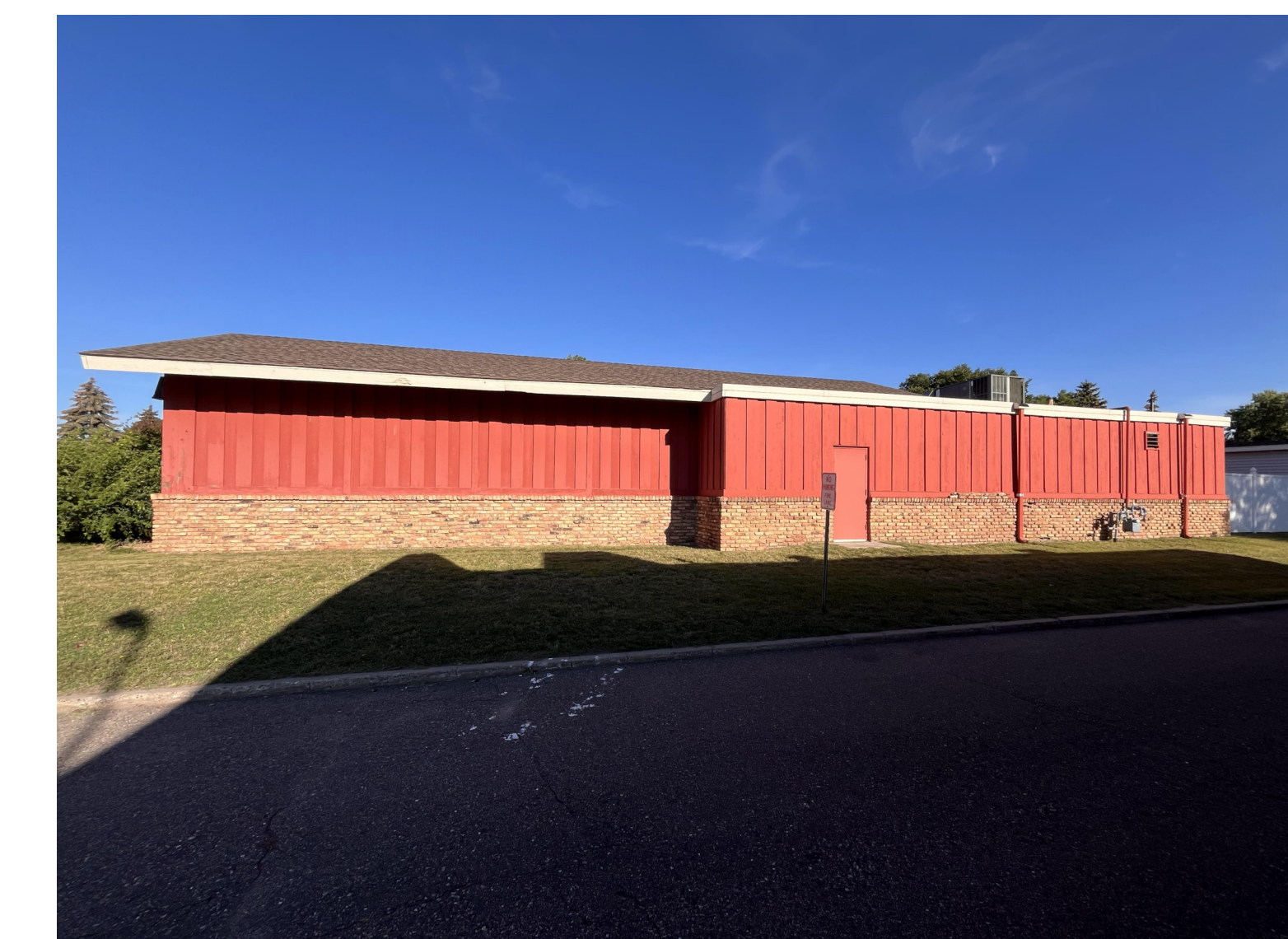
3 Existing Conditions SW
