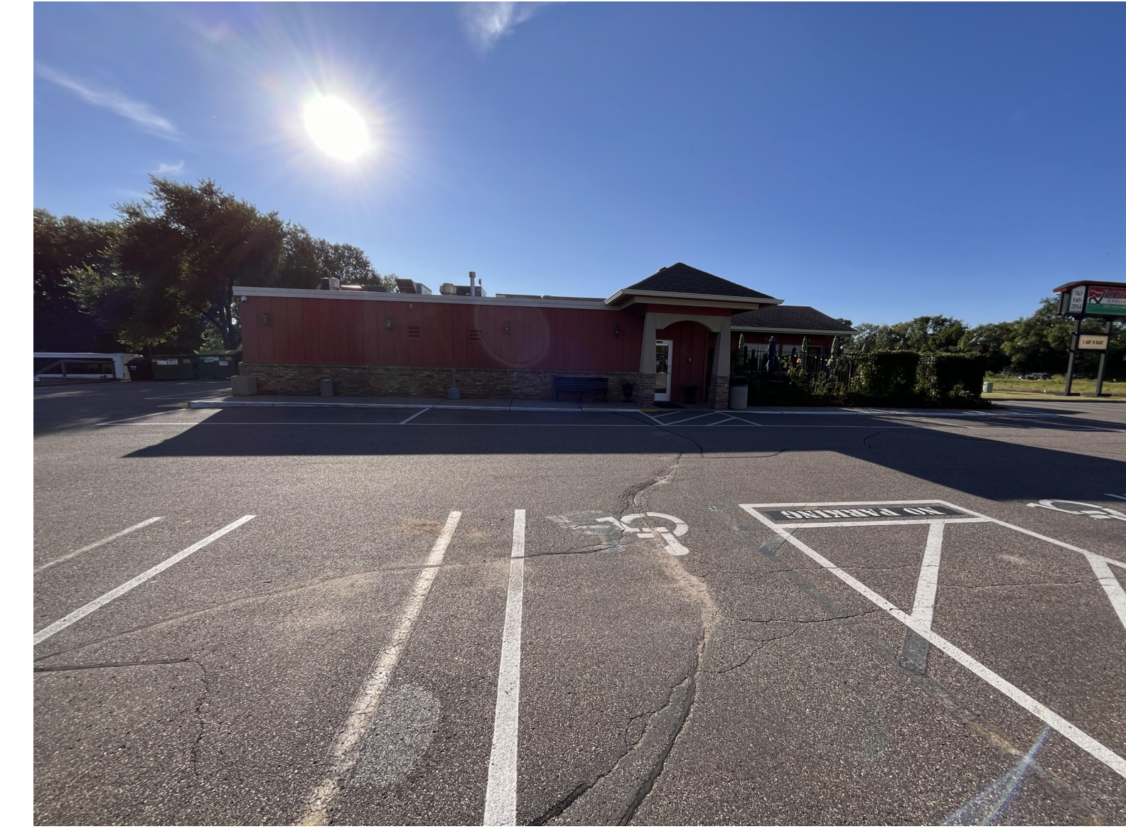
1 Existing Conditions NW
