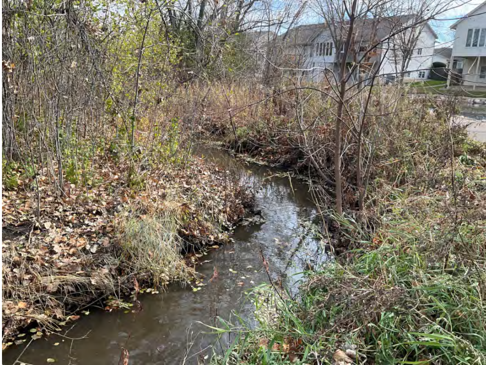
Photo 7: Site 1d. Looking downstream at station 7+75, the right bank is eroding due to a sharp turn and could encroach on the trail.
